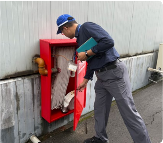
TSMC conducts supplier fire safety inspections.
