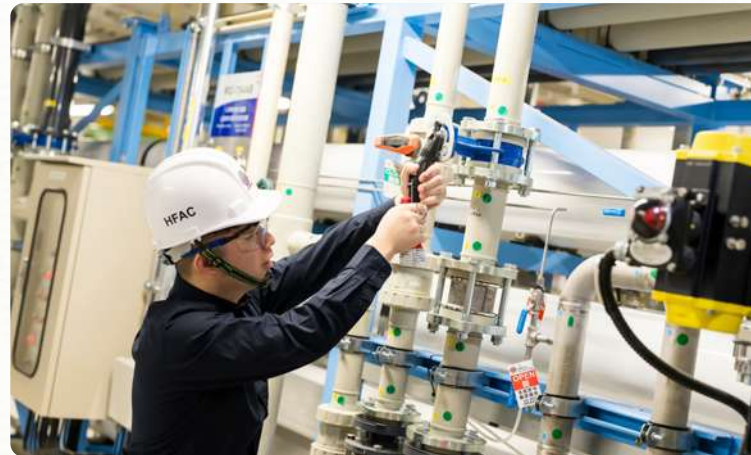
TSMC conducts NH 4 -N wastewater separation based on the concentration to improve treatment efficiency.
