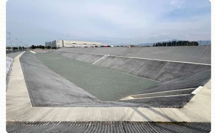
Conservation pond of the water conservation engineering at JASM.
