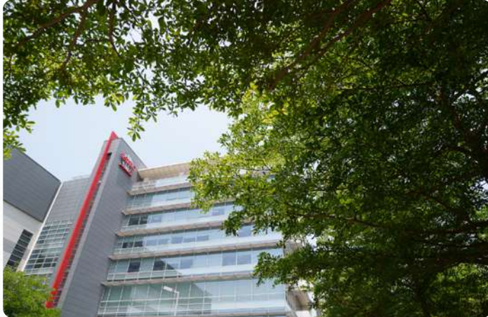
TSMC introduces reclaimed water into fabs with advanced processes.
