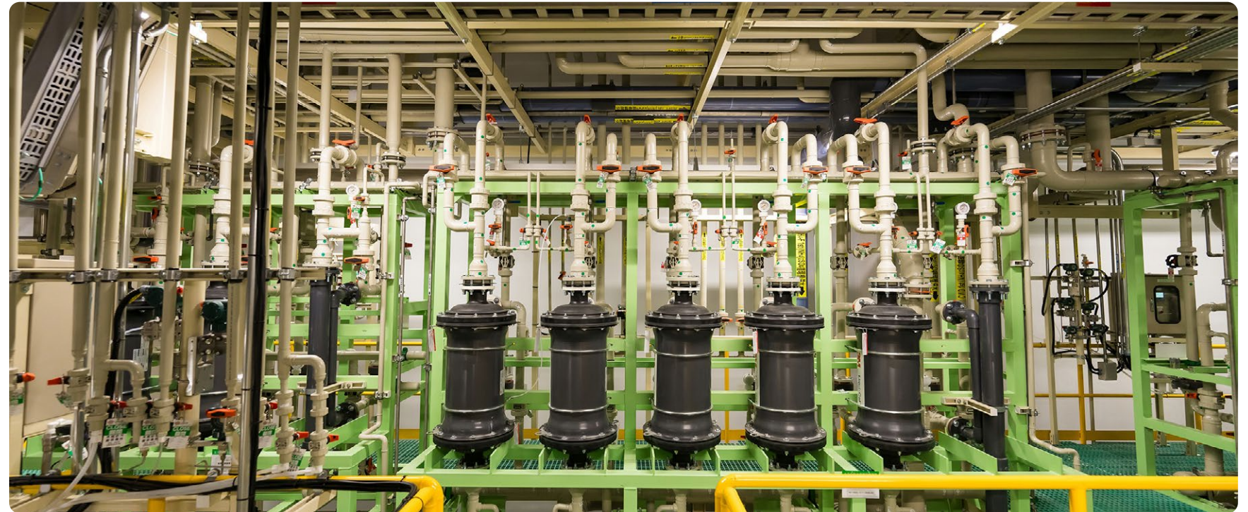
▲ TSMC optimizes its ammonia nitrogen wastewater segregation and treatment system, lowering environmental impacts.
