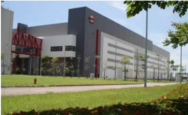
TSMC Fab 14 P3 Green Building
