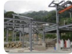
Main structure of the Lijia Bamboo Shoot Processing Plant completed
