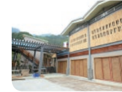
Construction on the Lijia Bamboo Shoot Processing Plant completed
