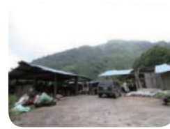
Surveying the site for the Lijia Bamboo Shoot Processing Plant
