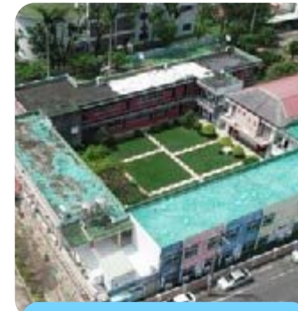
Before installation of solar panels
