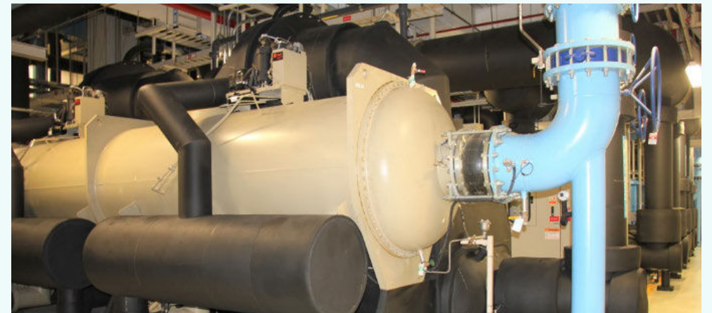
TSMC optimizes energy efficiency of water chiller systems through machine learning methods
