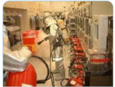
Emergency response drill - fire fighting
