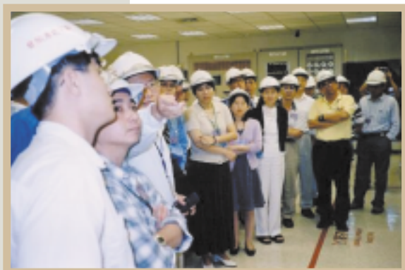
Control Center (Co-gen power plant of Hsin Yu Energy Development Co., Ltd.)
